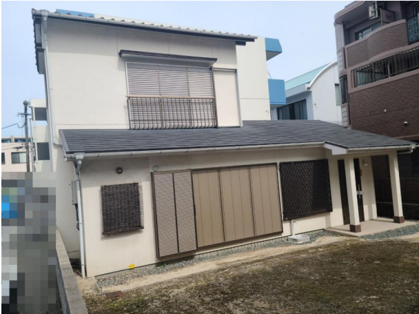
[外観・現況][現況写真]現地1
